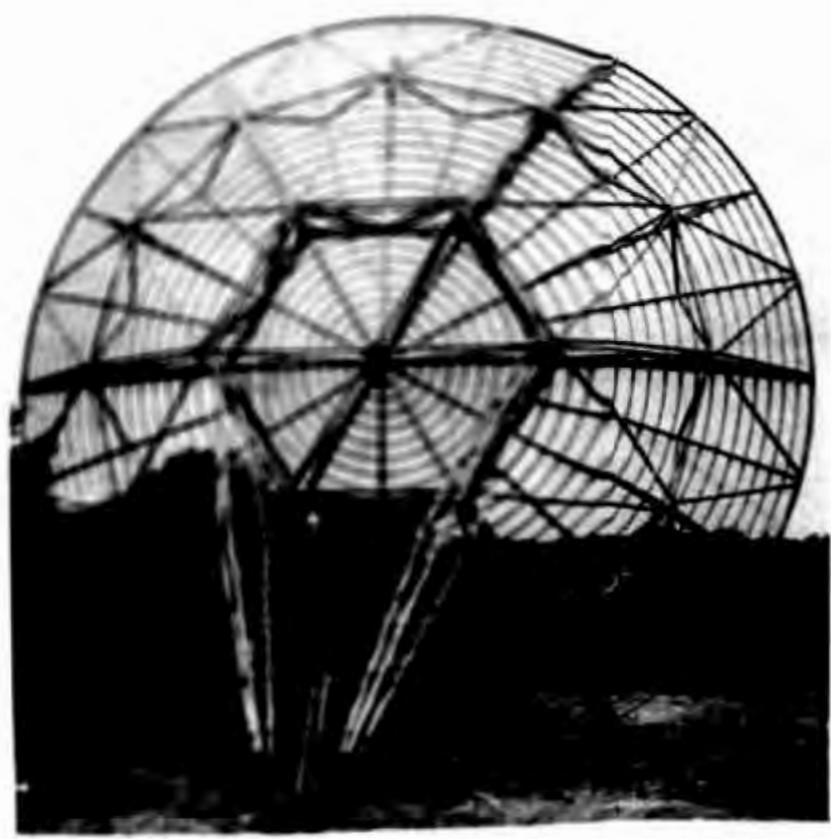
Fig VI-14 Twenty-eight foot paraboloidal antenna.
